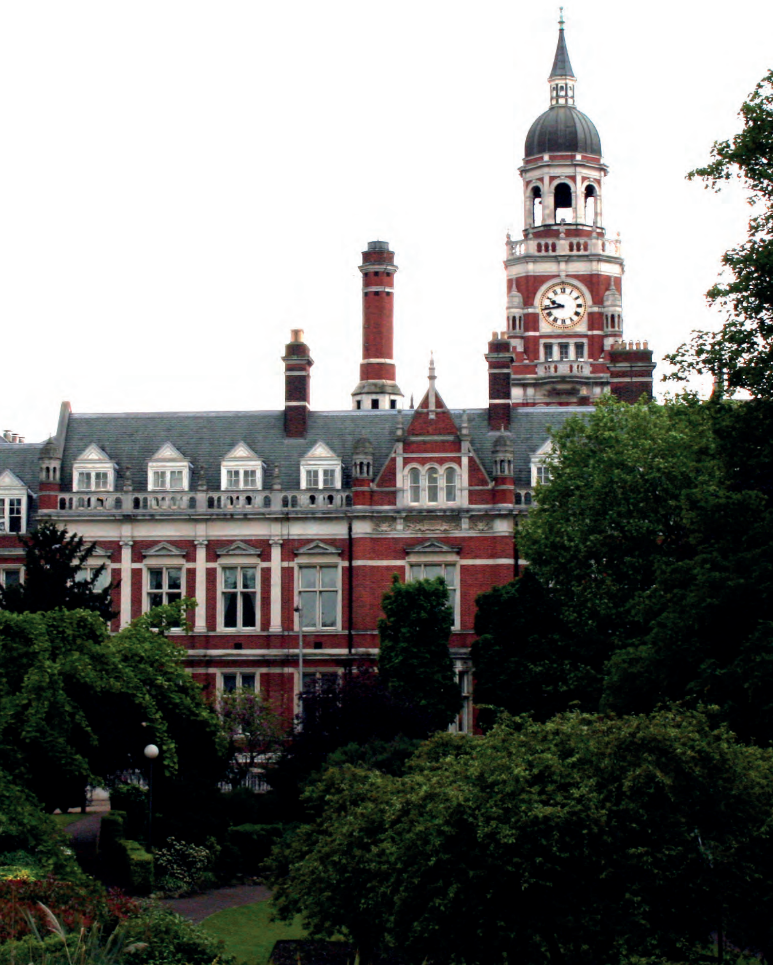
CROYDON TOWN HALL London - UK 2x KAPPA V EVO 51.2 - supply 1.100 kW
